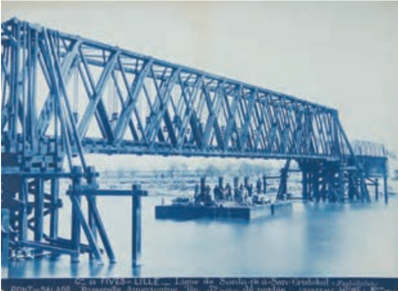
Construction Of The Railway Line Between Santa Fe And San Cristobald, 1890
