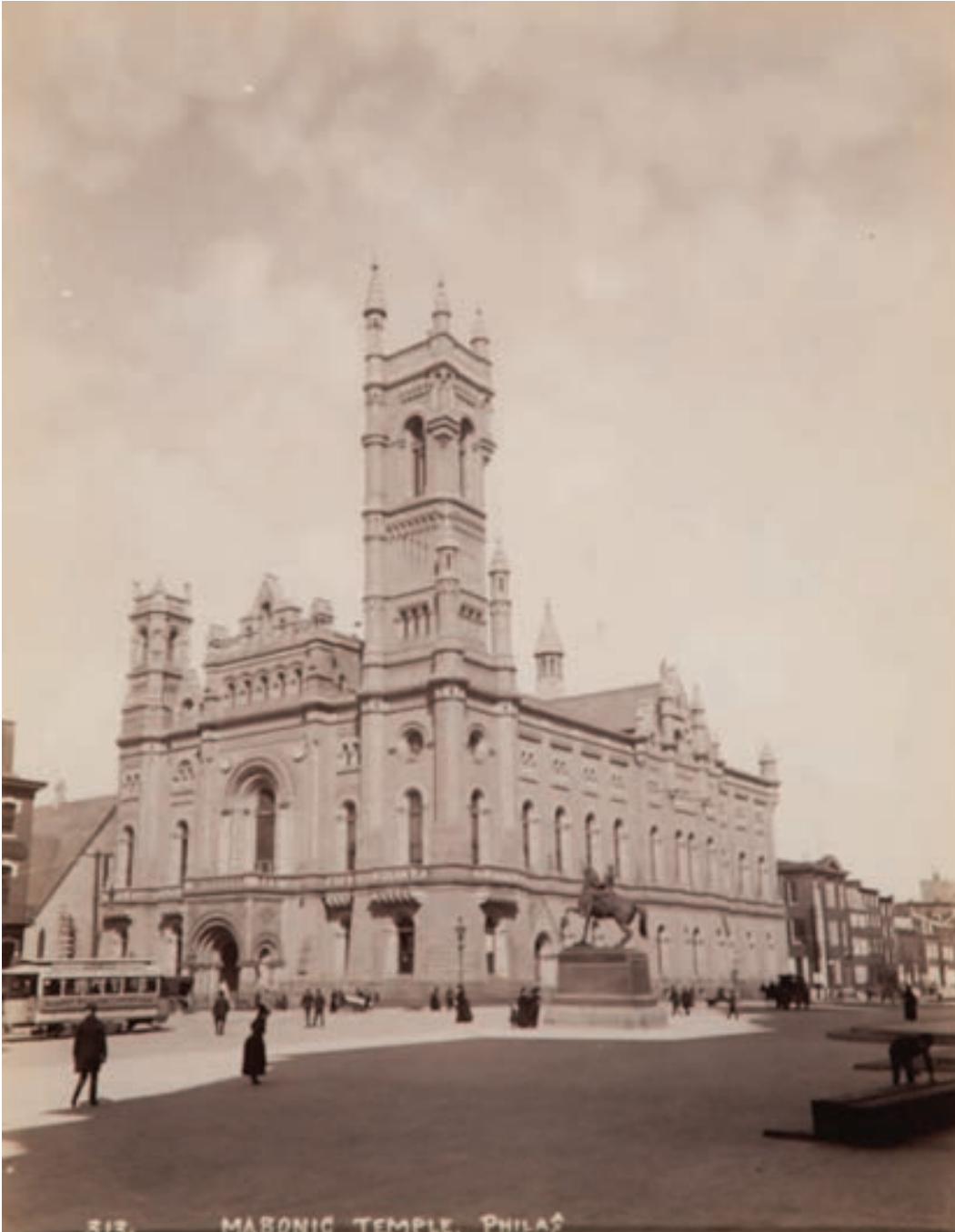
Philadelphia, Masonic Temple, after 1873 Unidentified photographer albumen silver print The Janos Scholz Collection of Nineteenth-Century European Photography 1981.031.075
